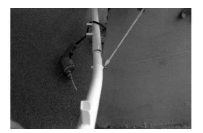
Use a 1/4" bolt to check the ends of the bushings. The head of the bolt should make contact all the way around. (See Standard Construction Procedures.)
